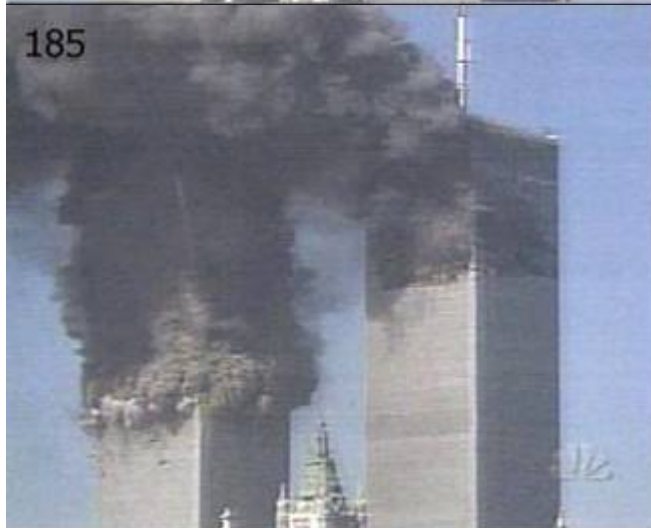
Figure 10: Pictures of WTC 2 at the time of collapse, showing frame numbers taken at 8 frames per second. There are 12 sec from the first to the last picture. Note the grey smoke coming from the floors below the initial fire.
