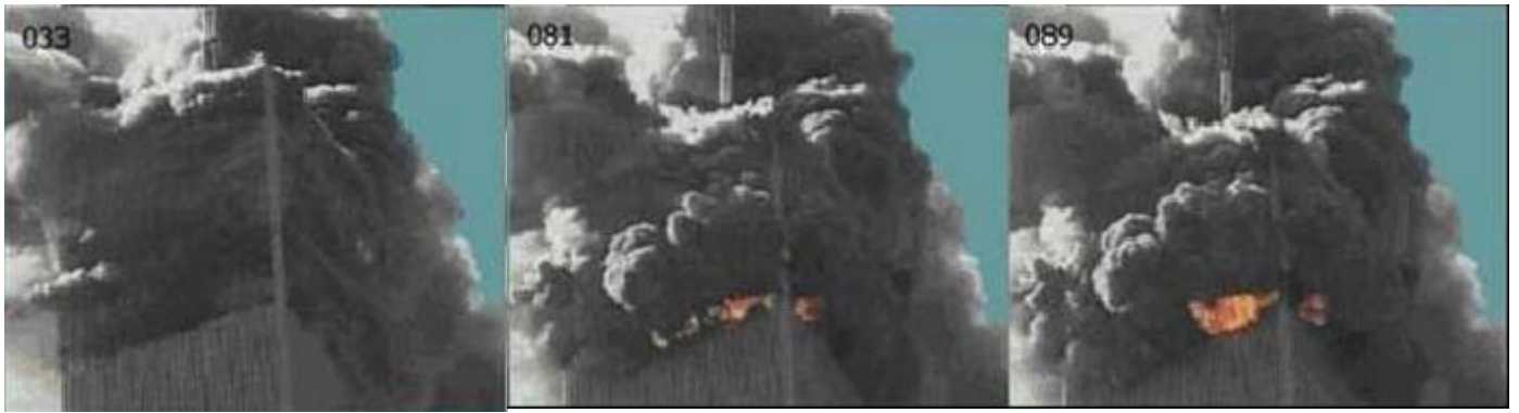
Figure 11 Pictures of WTC 1 at the time of collapse, showing frame numbers taken at 8 frames per second. It is 7 sec from the first to the last picture. Note the red fire spikes coming from the floors below the initial fire.
