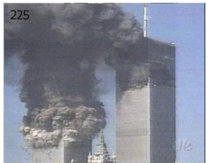
Figure 10: Pictures of WTC 2 at the time of collapse, showing frame numbers taken at 8 frames per second. There are 12 sec from the first to the last picture. Note the grey smoke coming from the floors below the initial fire.
