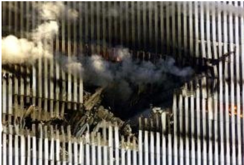
Figure 4: Picture of WTC 1 immediately after the airplane had cut its way into the building 8 . The contour of the airplane is visible.
