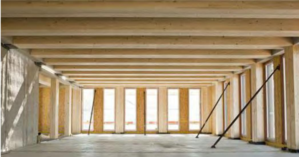
New technology in post and beam construction includes the use of post-tensioned cables for additional strength and stability. This technology is commonly known as post-tensioned timber construction and is discussed below.
