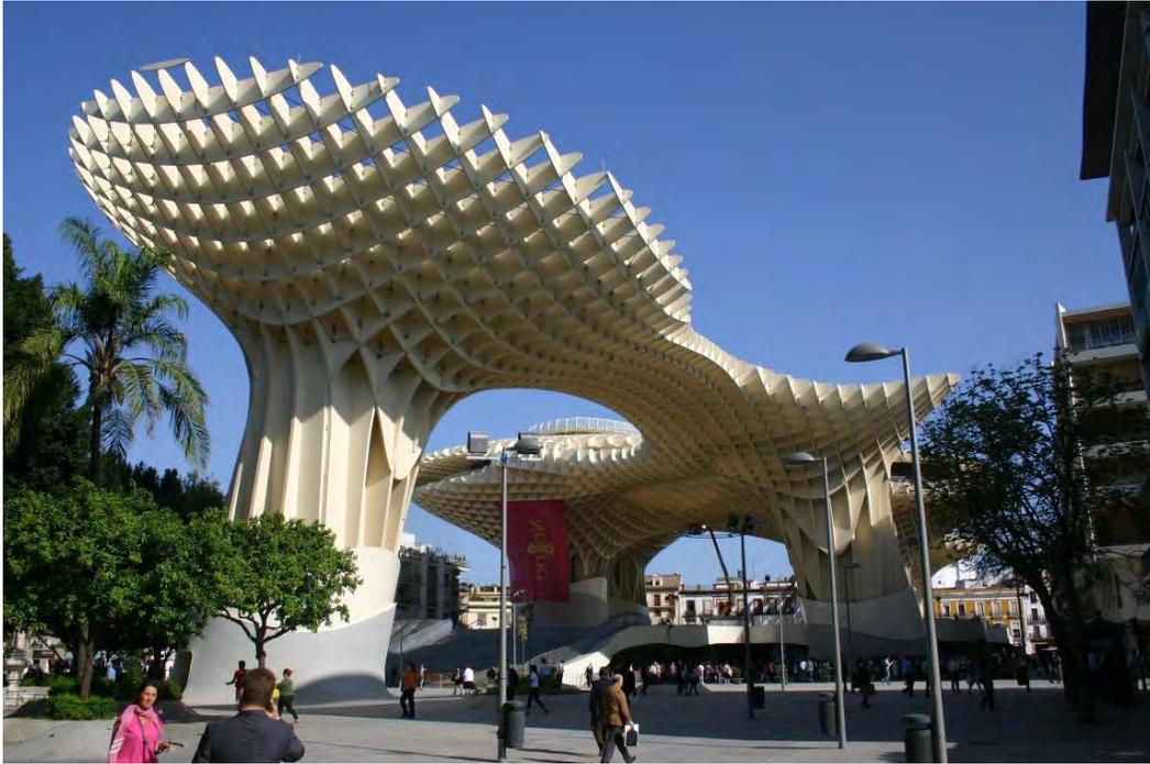
The structure is composed of micro-laminated timber sections protected by a waterproof polyurethane coating. Structural elements are connected by over 3000 connection nodes at the intersection of timber elements (Arup, 2012).
