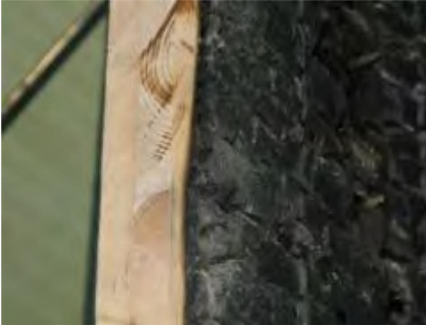
Despite the inherent fire resistance of heavy timber CLT panels, CLT elements are often required to be encapsulated by non-combustible gypsum board protection. This is intended to protect exposed CLT panels from heating and combustion and increase the fire resistance rating of the structural assembly. An example of gypsum board protection for a CLT wall is shown in the figure below.
