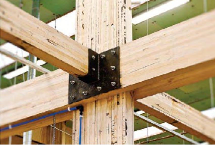
Figure 29 – Glulam beams (APA, Engineered Wood Construction Guide: Glulam, 2011)
