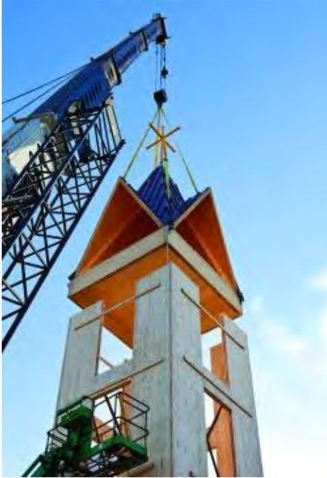
Recognized as the first structure in the US to be built in CLT, the 78 foot tall [24m] bell tower at the Myers Memorial United Methodist Church in Gastonia, North Carolina was completed in 2011 (Thatcher, 2011).
