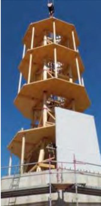
Completed in Hannover, Germany in 2012, TimberTower is a wind turbine constructed of glulam prefabricated panels that were assembled onsite (Quick, 2012).
