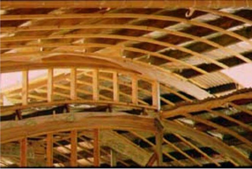
Figure 31 – LVL roof beams (WoodSolutions, Laminated Veneer Lumber (LVL), 2013)
